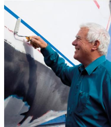
In order to keep a paint system in good condition, the system needs to be maintained from time to time by applying one or more maintenance coats. If the existing paint work is still intact and only shows discoloration or loss of gloss, degrease the surface with Epifanes Spraythinner for Paint & Varnish or denatured alcohol, sand with 220 dry and apply one or more maintenance
